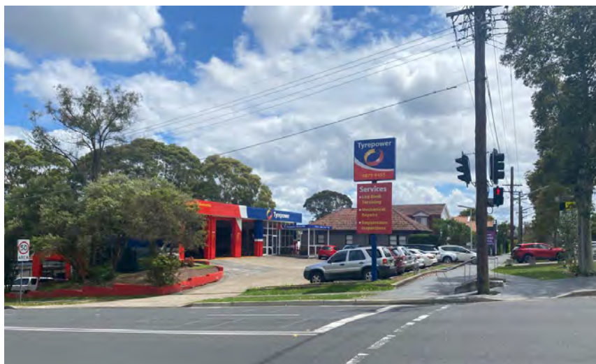
Figure 12: 142 Pittwater Rd, located on corner of Pittwater Rd and Thompson St within B1 zone under RLEP 2014. Source: CPS – Site Inspection, 16 January 2023.
