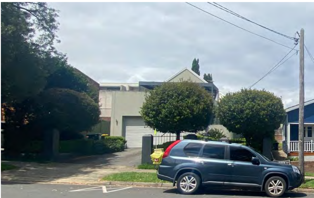
Figure 5: 57 Thompson Street as viewed from Thompson Street looking south towards the site. Source: CPS – Site Inspection, 16 January 2023.
