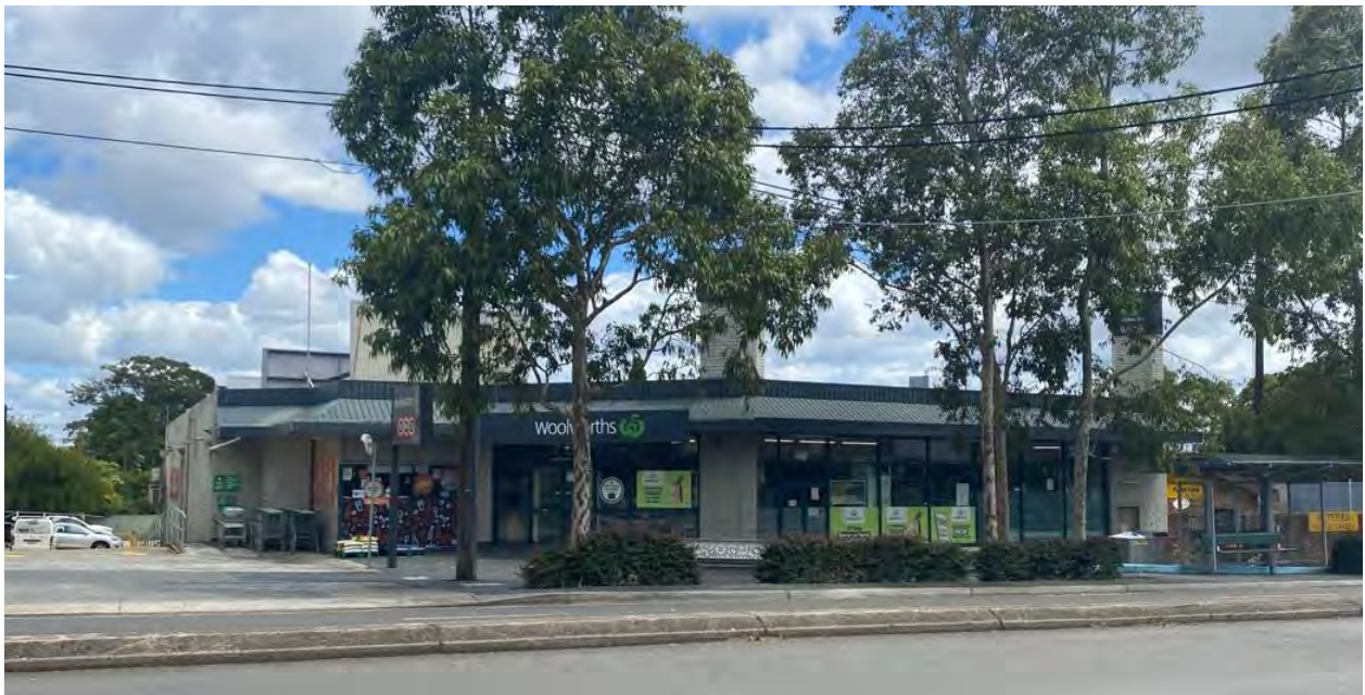
Figure 3: 130 Pittwater Road as viewed from Pittwater Road looking west towards the site. Source: CPS – Site Inspection, 16 January 2023.
