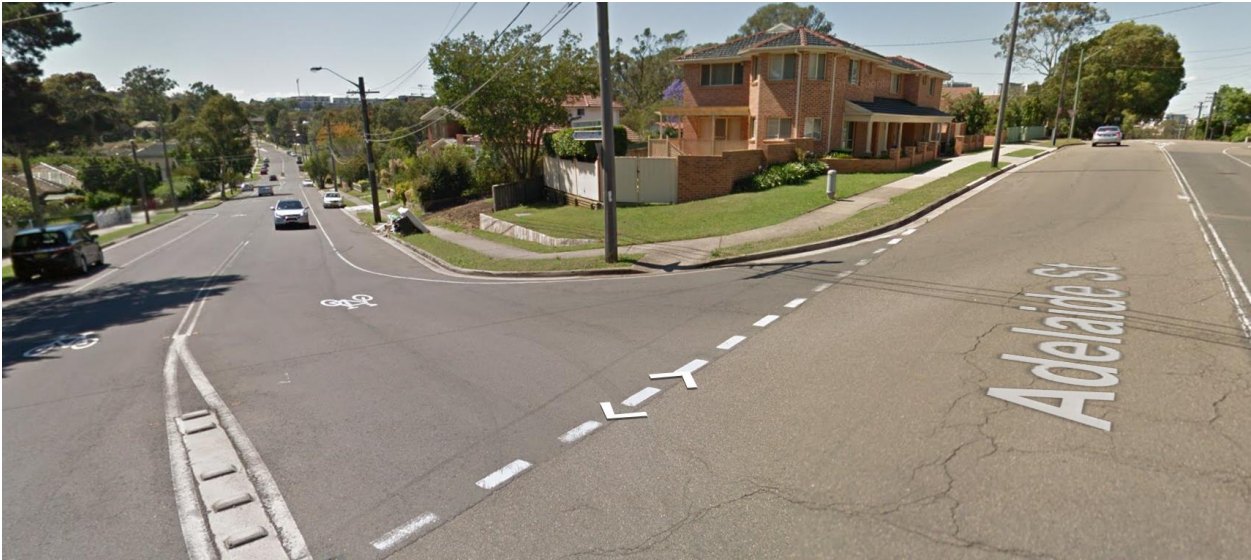
Figure 1 Residents property on the corner of Adelaide St and Constitution Road West
