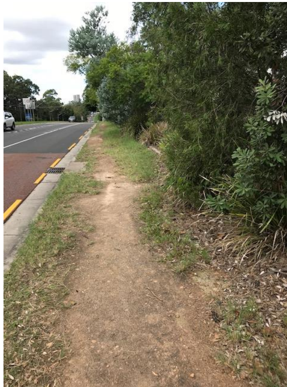
Figure E2: Existing footpath and road configuration in Epping Road, adjacent to Yarwood Street
