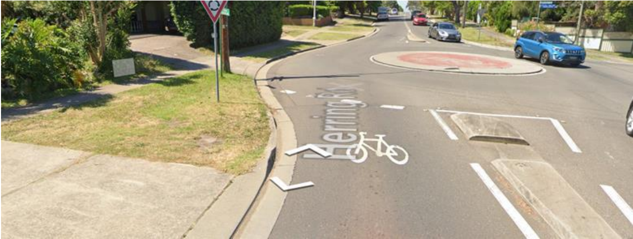
Figure 2: Missing Kerb Ramp on Herring Road
